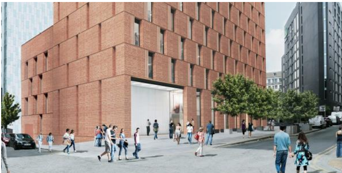
Main entrance off Hulme Street including patter brick work to Great Marlborough Street
